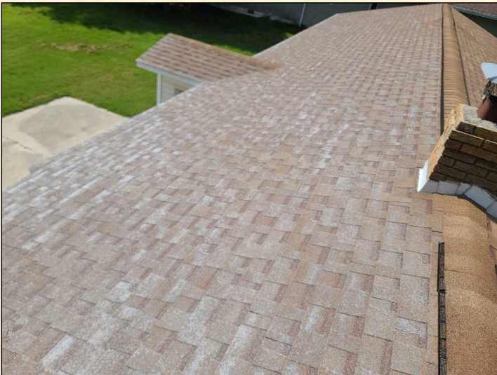
Extensive granular lost noted with numerous tabs having almost complete granular loss.
