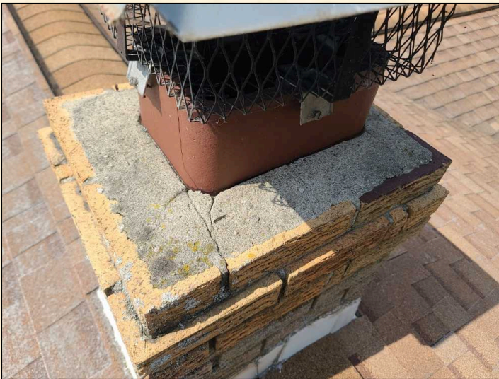
Brick and mortar deterioration observed; repair advised.
