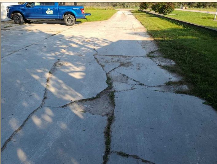
Grounds Driveway and Walkway Condition
