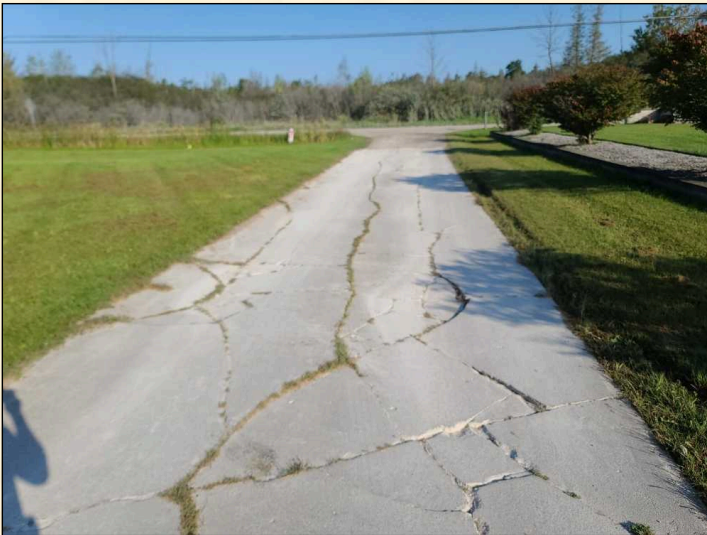
Grounds Driveway and Walkway Condition
