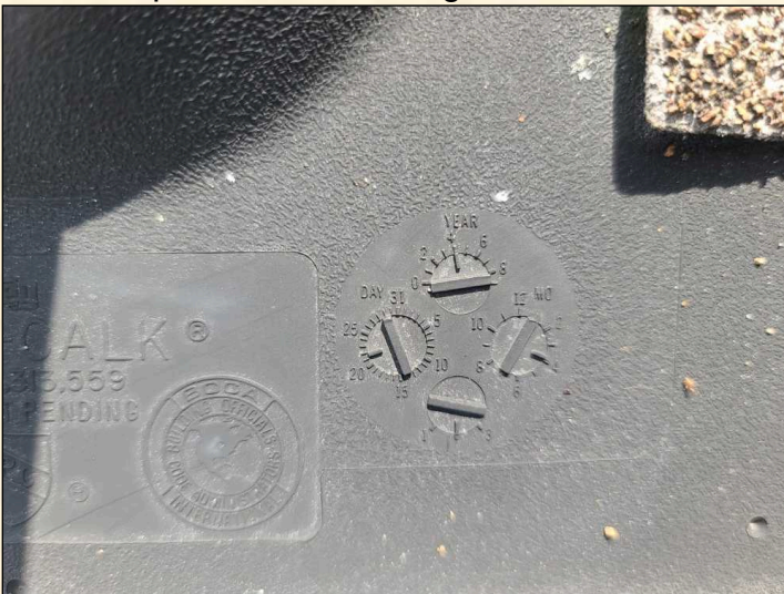
Vent boots from 2004. Estimated roof age
