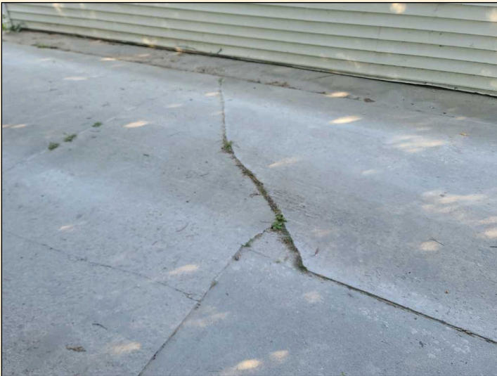
Grounds Driveway and Walkway Condition
