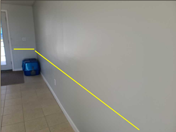
Interior Areas Wall Condition
