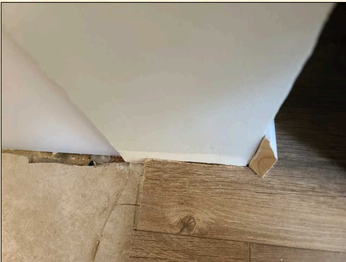
Interior Areas Floors
