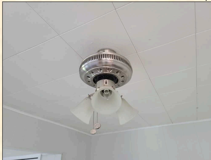
The ceiling fan is missing blades, generic replacement blades are available at your local home improvement center.
