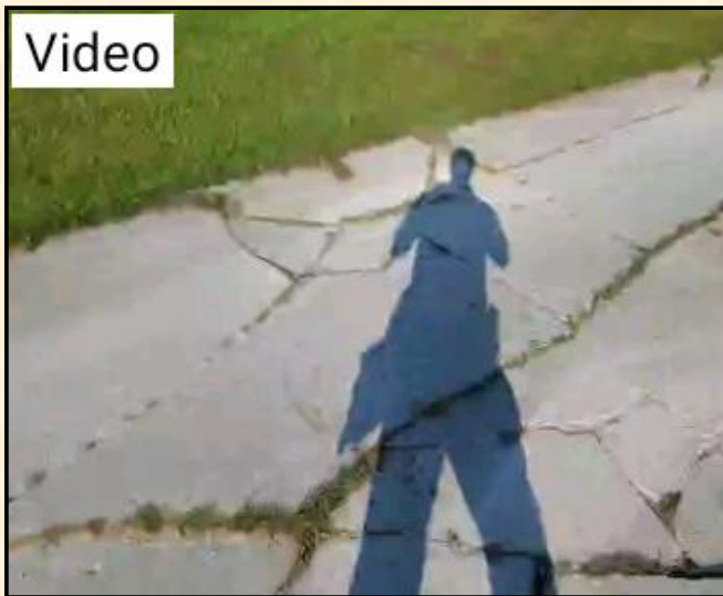
Grounds Driveway and Walkway Condition
